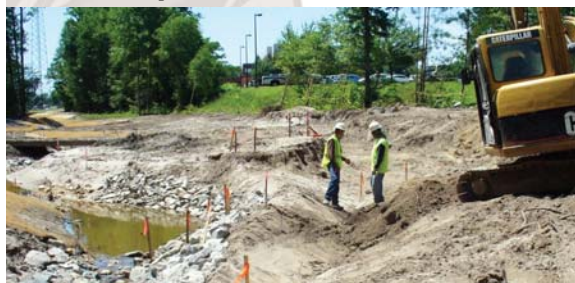
Crews worked to reconnect the Rocky Branch stream to the floodplain and replant native vegetation on its banks as part of a stream restoration project in FY 09.
